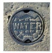
Fig. 22. Typical municipal water system supply valve cover in Oak Park. (photo by M. Iversen)
